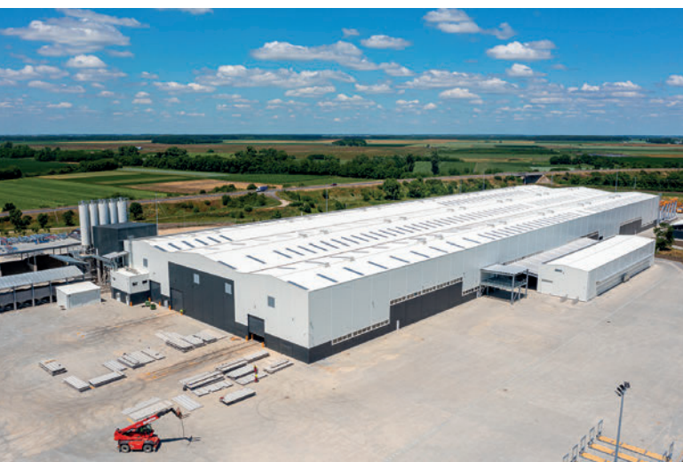
Viastein Kft belongs to the Bayer Construct group and is one of the biggest precast plants built in Hungary.
