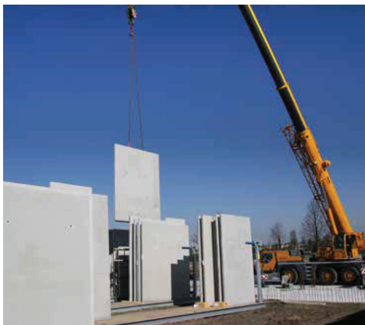
Kaczmarek primarily uses the double walls and lattice girder floors to construct residential buildings, which can be supplied quickly, sustainably and cost-effectively
