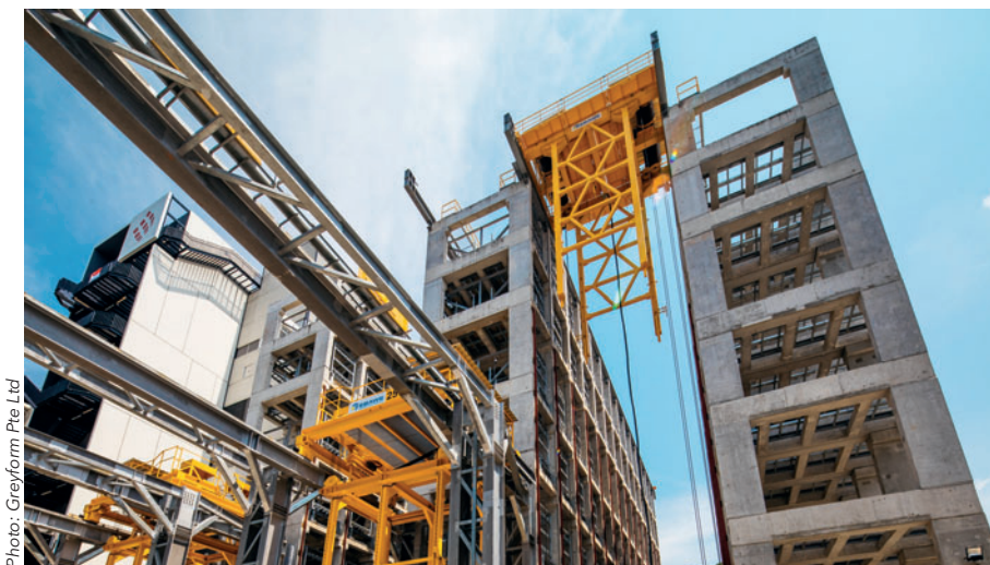
Because of the demands on limited space, the warehouse has not been constructed horizontally, but vertically. The precast concrete elements are stored fully automatically on complete racks on one of the 7 levels and withdrawn again as required.
