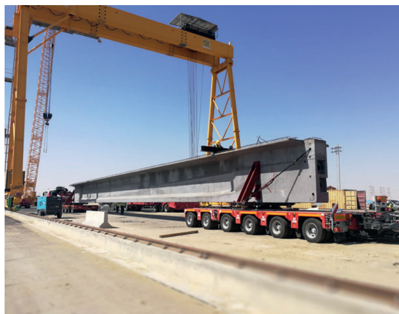
Due to the convenient location of the production yard, which is placed in the middle between the 2 furthest construction sites, the transport ways have been minimized to 20 km max.
