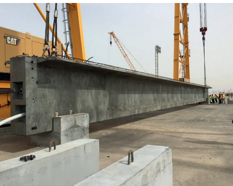
The elements are produced post-tensioned. Eight elements can be produced daily. For all bridges a total of 820 girders are required.
